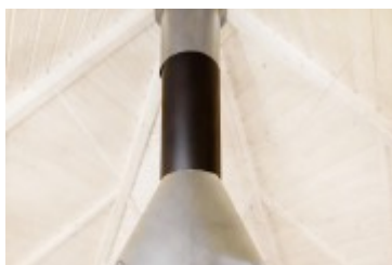
Grill Chimney Extension
